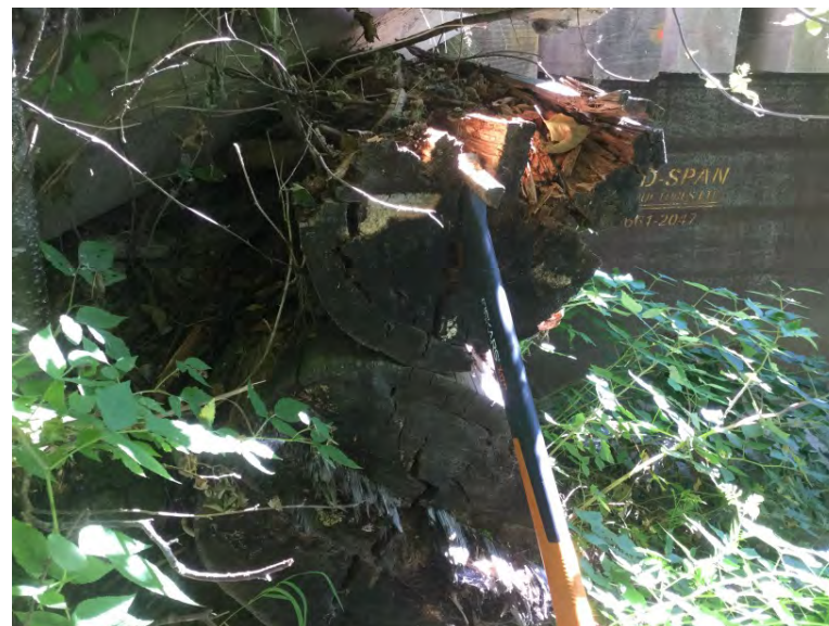
Ballast wall condition for steel girders
