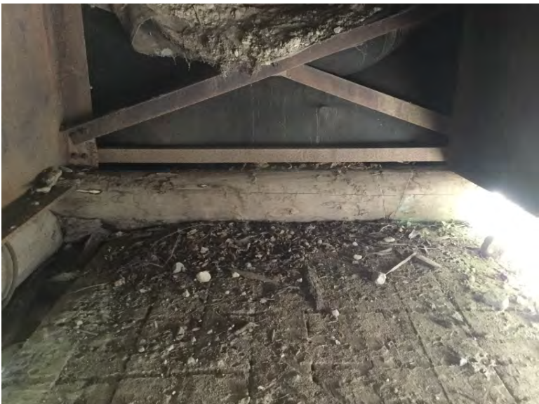
Right bank sill for steel girders
