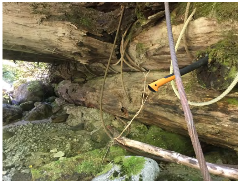
Left Bank Abutment when facing downstream
