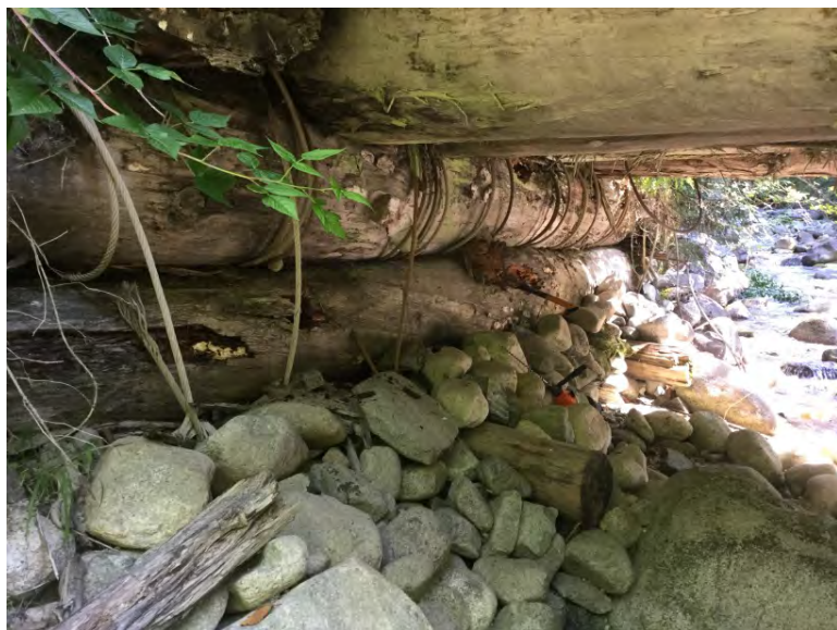
Right Bank Abutment when facing downstream
