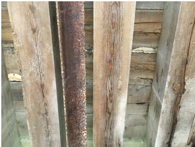
Timber deck condition
