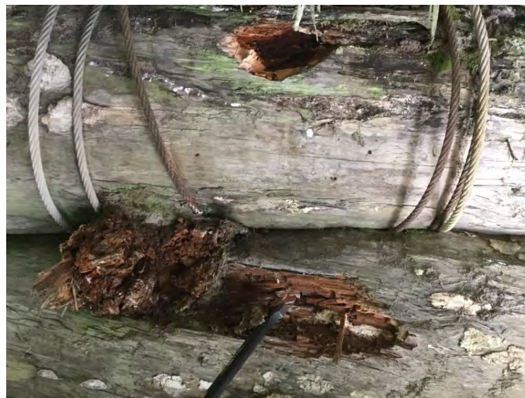
Right Bank Abutment when facing downstream
